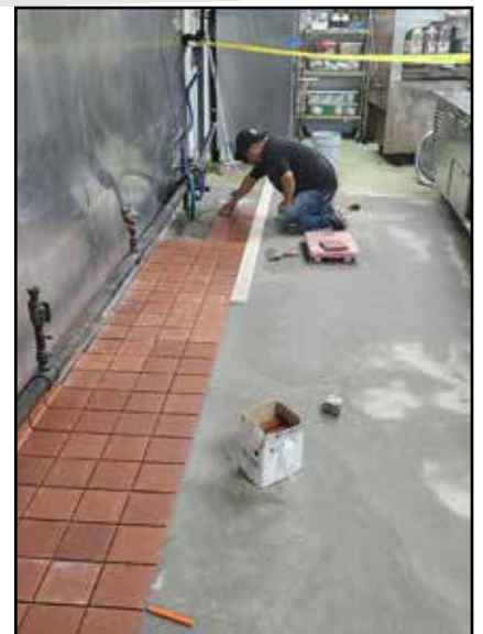
New Hot Line Floor
